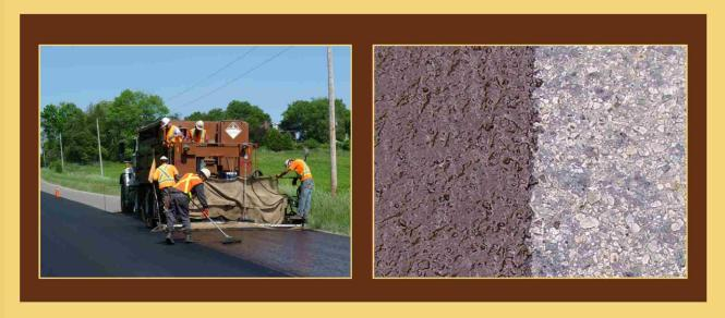
It is a thin surface treatment not appropriate to resolve pavement structural deficiencies. These systems are well suited as a preventive maintenance treatment to extend the life of sound, low traffic volume pavements. Preventive maintenance treatments are low-cost treatments that retard deterioration of the pavement, maintain or improve the functional condition of roadways, and extend the pavement's service life when applied to suitable candidates.
